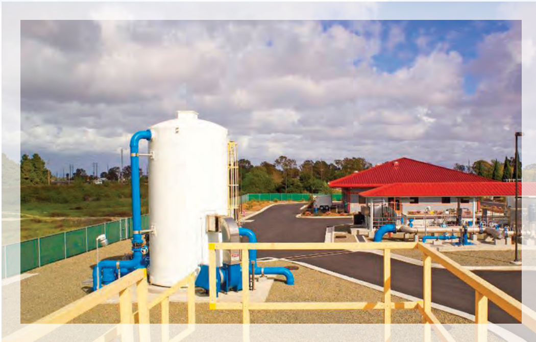
Leo J. Vander Lans Advanced Water Treatment Facility in Long Beach, California
