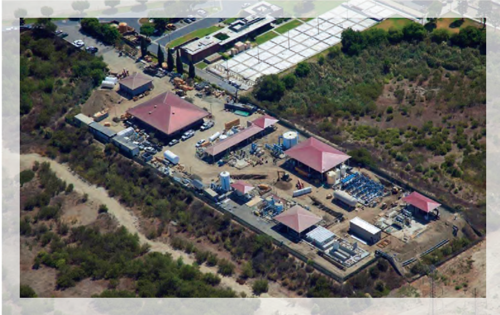
Leo J Vander Lans Water Quality Treatment Plant
