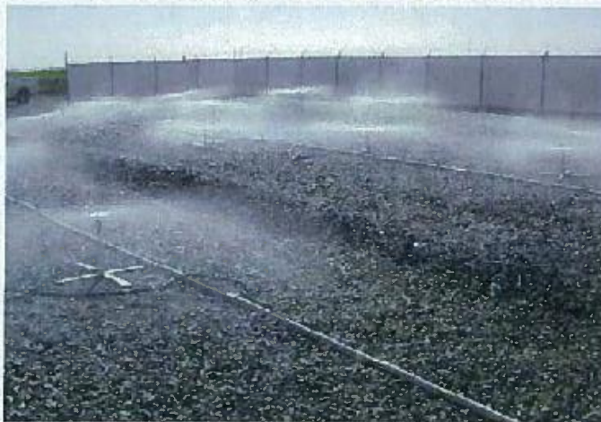
Drain water being applied to a gravel bed collector in a solar evaporator (vertically oriented nozzles at riser height = 1.00 ft)
