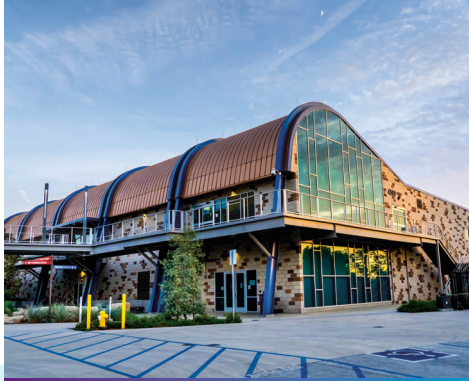
WRD's advanced water treatment facility at the Albert Robles Center in Pico Rivera.
