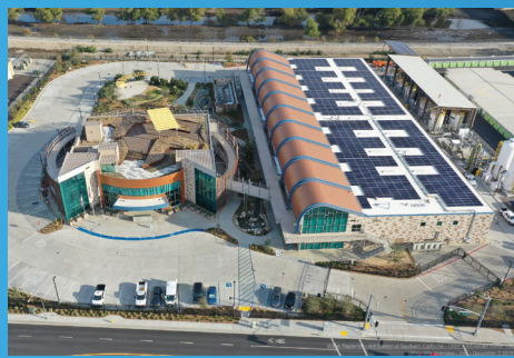
Aerial view of ARC's advanced water treatment facility, learning center, sustainable gardens, and solar panels.
