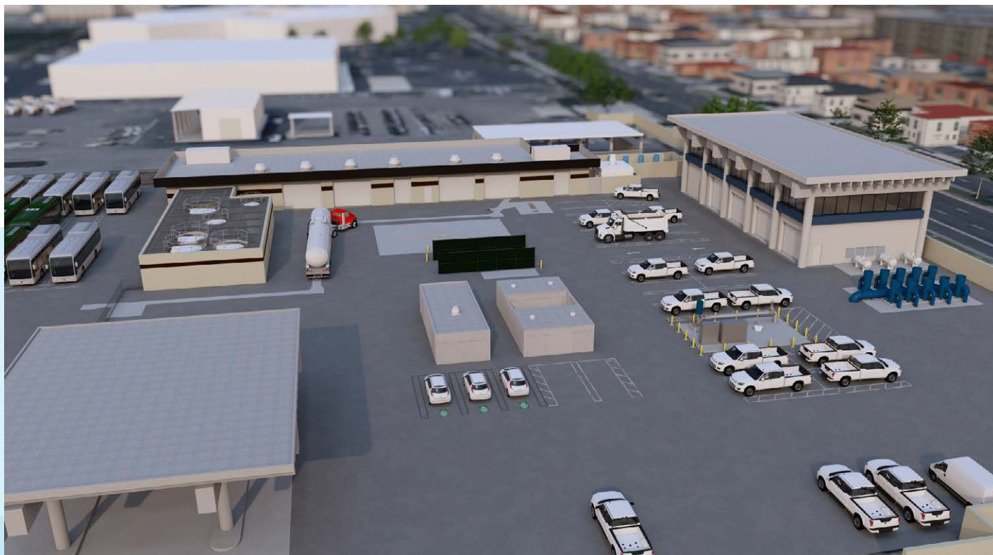
An early rendering of what the expanded Torrance Groundwater Desalter may look like. The expanded facility will include additional pretreatment, reverse osmosis, and automated strainers to protect the reverse osmosis systems.
