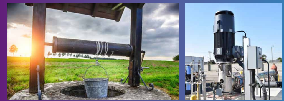
Modern groundwater wells are motorized pumps that can access multiple aquifers at once. There are over 300 of these 'production wells' in the WRD service area.
