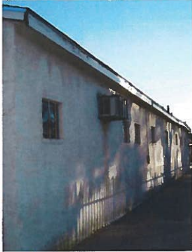
1947 building: View looking southeast at the west elevation
