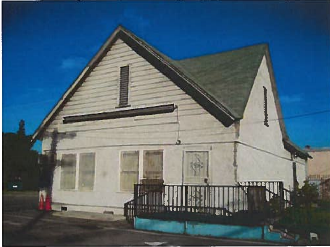
1913 building: View looking northeast at the west and south elevations
