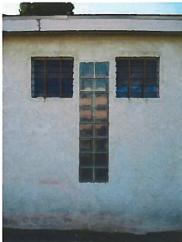
1947 building: Detailed view looking west at the east elevation
