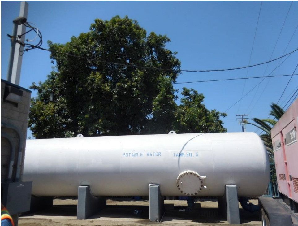
Photograph 1. View of existing hydropneumonic surge tank facing north.
