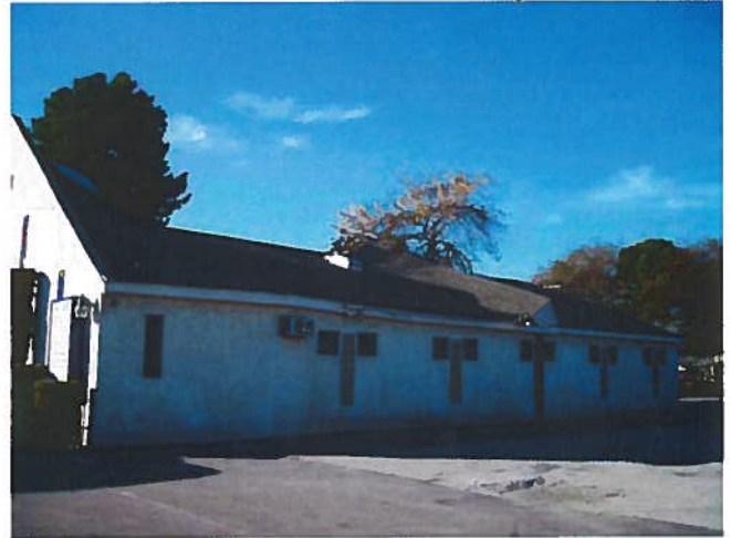
1947 building: View looking northwest at the east elevation
