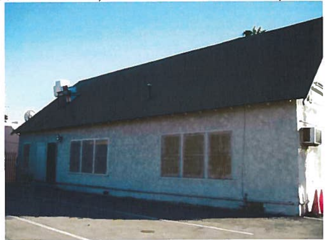
1913 building: View looking southeast at the north elevation
