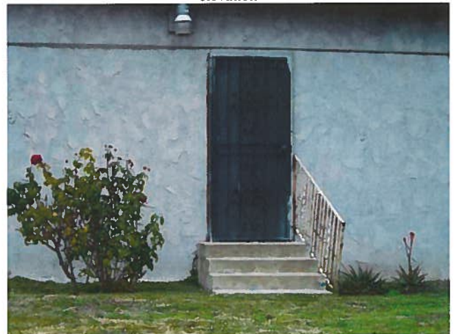
1913 building: View looking north at the entrance at the south elevation
