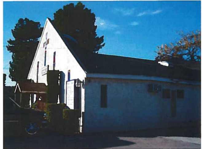
1947 building: View looking northwest at the south section of the east elevation, and the façade
