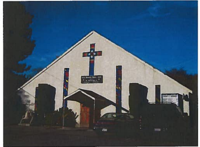
1947 building: View looking north at the façade
