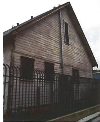
1913 building: View looking northwest at the east elevation
