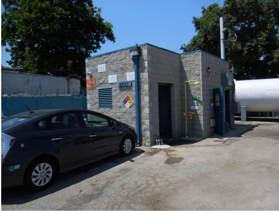
Photograph 3. View of gas chlorinator facilities facing north.
