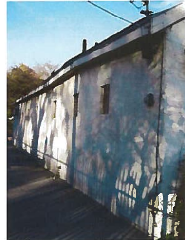
1947 building: View looking northeast at the west elevation
