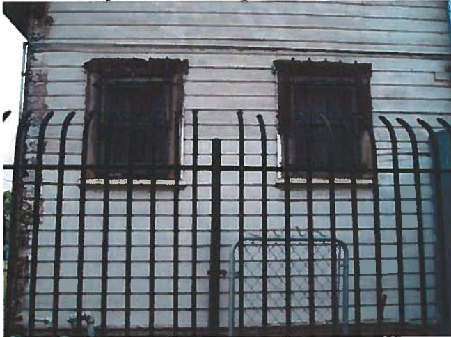
1913 building: View looking west at the windows at the east elevation
