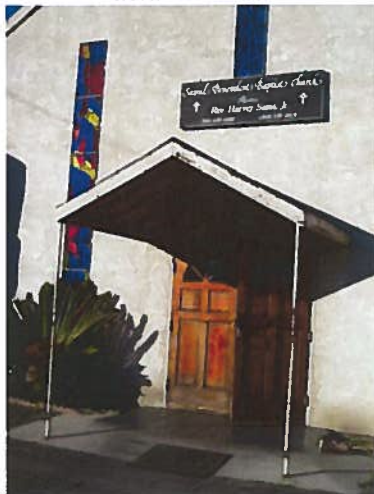
1947 building: View looking northwest at the primary entrance
