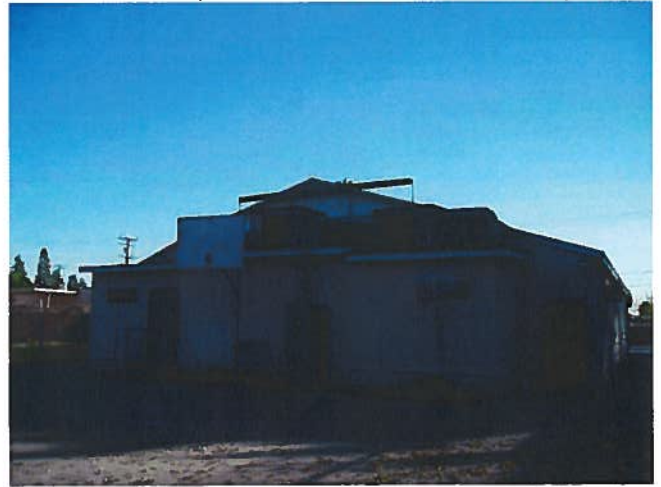
1947 building: View looking southeast at the north elevation; the basketball court is in the foreground
