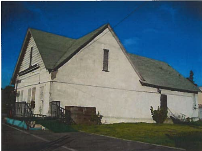
1913 building: View looking northeast at the south and west elevations
