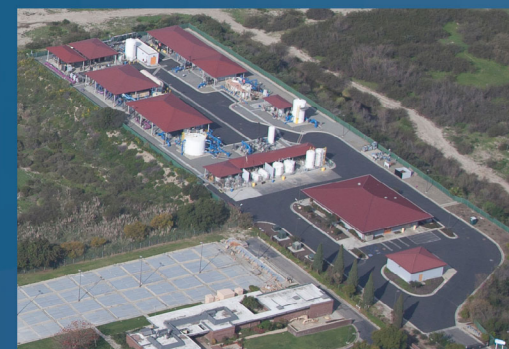
Leo J. Vander Lans Advanced Water Treatment Facility
