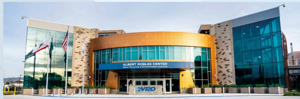
Rain or shine, WRD recycles 14.8 million gallons of water per day at the Albert Robles Center
