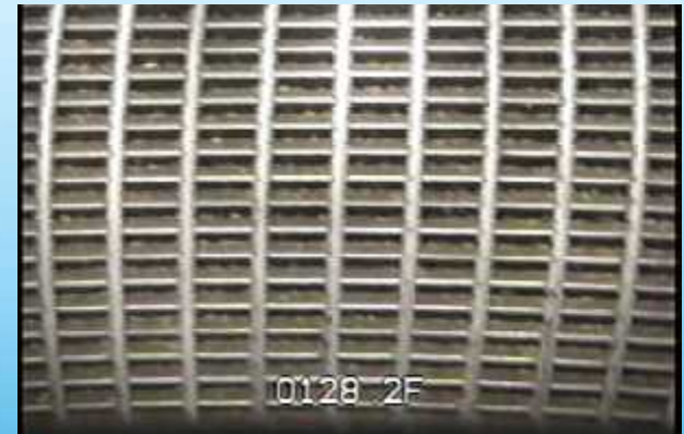
Cleaned Well Screen and Gravel
